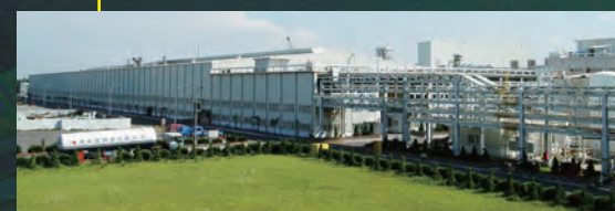
▲ CARBON FIBER PLANT IN MAILIAO COMPLEX
